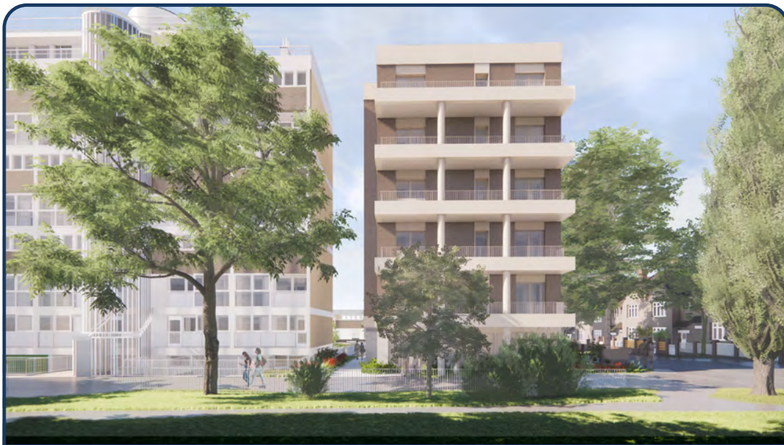
① View over Highgate Enclosures of Haddo House and the new homes from Highgate Road
