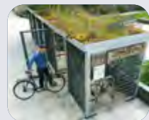
Green roofed storage
